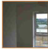
Putty finished interior walls with plastic emulsion paint
